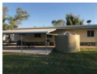
New staff kitchen/dining room
